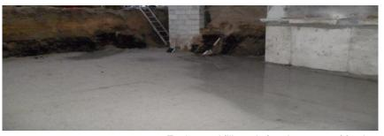
Engineered fill ready for placement of footings.
